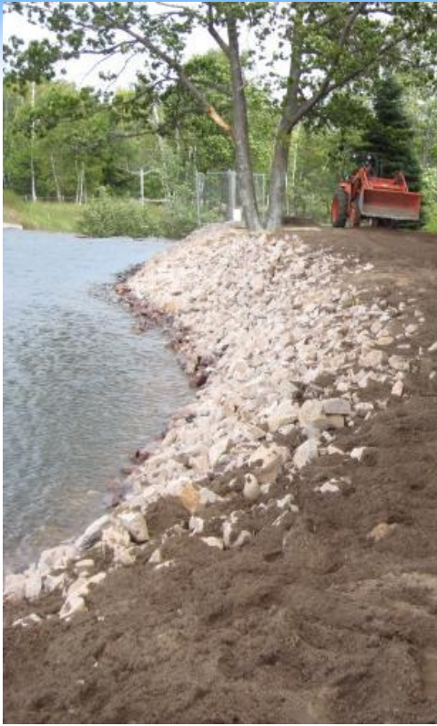
Left: Completed bank structure consisting of sand, rock, and top soil.
