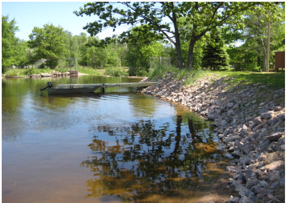
The following spring the bank was visually appealing and permanent. Note the grass growing between the rocks and the clarity of the water seen in the reflection of the tree..
