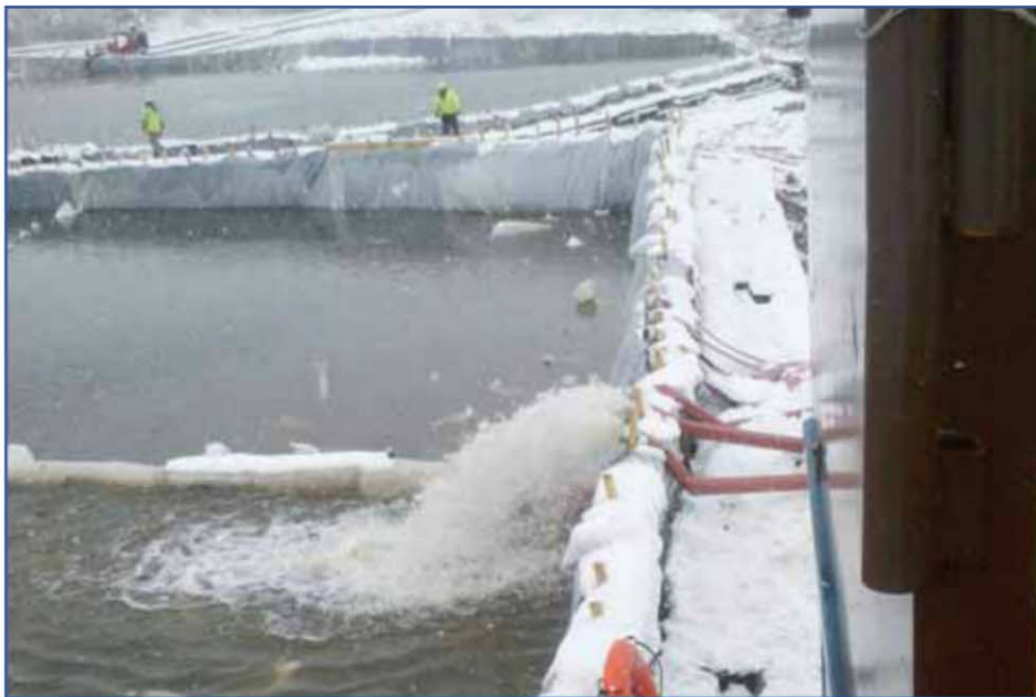
4 lines opened for flood control.
