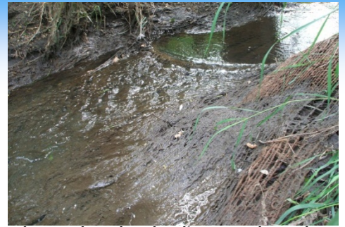
Above: Flocculated sediment and metals attached to jute matting result in clear water discharging from the treatment train.
