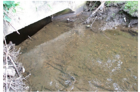
Above: Success is evident with clear water exiting.
