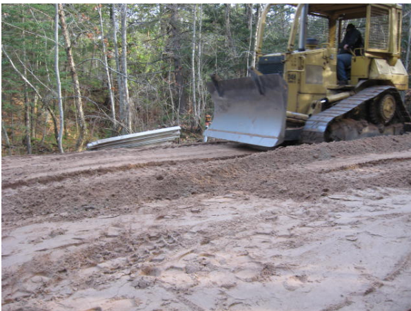
After the box culvert was finished, the backfilling, grading and compaction had to be done for the preparation of the new road surface.
