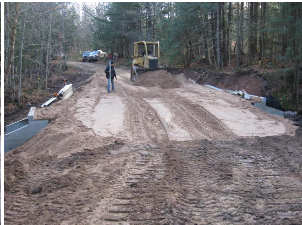
After the box culvert was finished, the backfilling, grading and compaction had to be done for the preparation of the new road surface.
