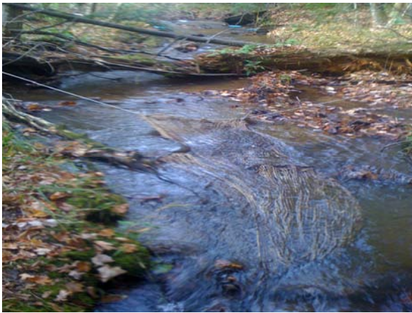
Floc Logs can be seen in the stream preventing turbidity migration.
