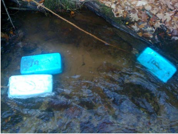
Floc Logs can be seen in the stream preventing turbidity migration.
