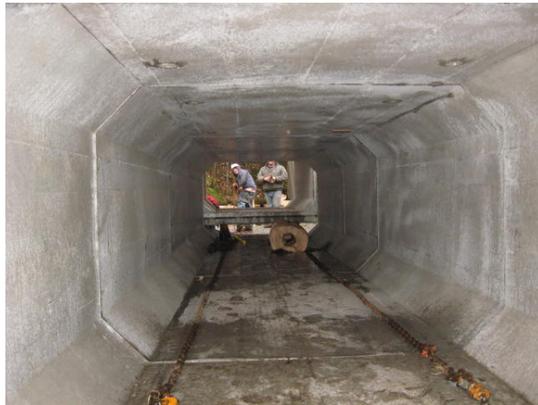
Looking through the culvert after all segments are assembled.
