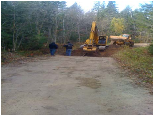
This is the beginning of the removal of the old culvert using an excavator.
