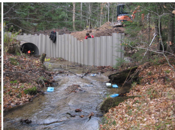
This is the beginning of the removal of the old culvert using an excavator.
