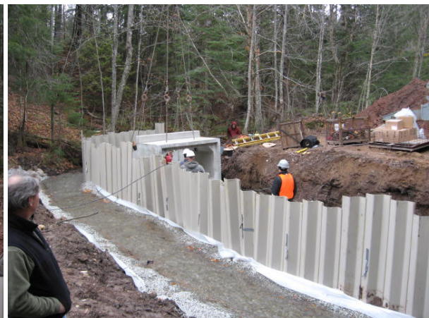
Placement and assembly of the new box culvert is in progress.
