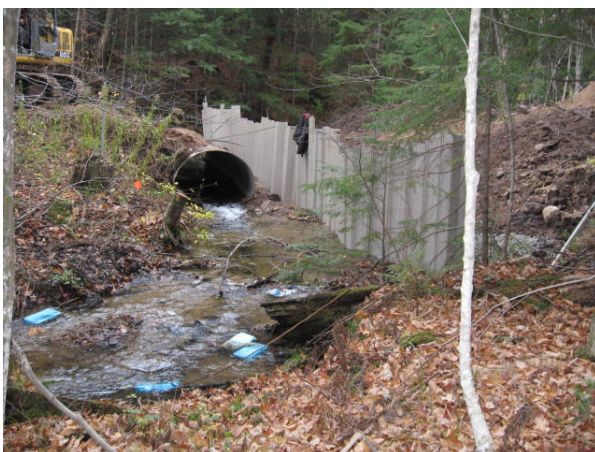
This is the beginning of the removal of the old culvert using an excavator.
