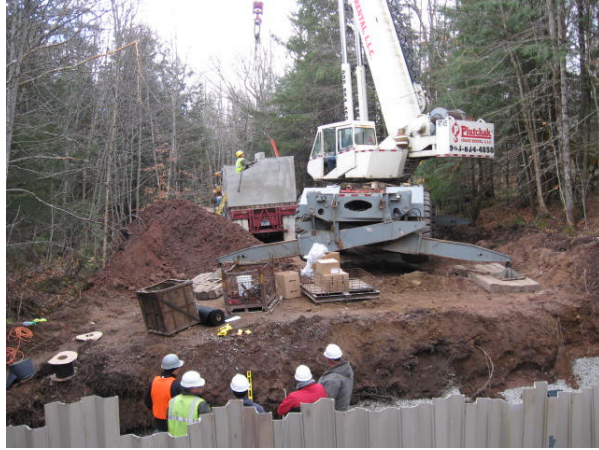
The installation of the new box culvert is beginning.
