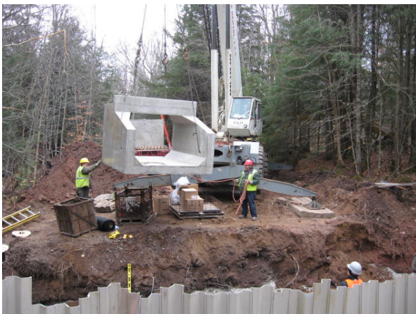
Placement and assembly of the new box culvert is in progress.
