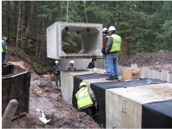
Assembly of the new box culvert is continued
