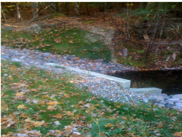
The polymer mixture was spread on all the soil that was disturbed. The polymer not only stabilized the soil but prevents the seed and fertilizer from washing into the stream.
