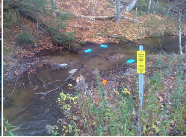
Floc Logs can be seen in the stream preventing turbidity migration.
