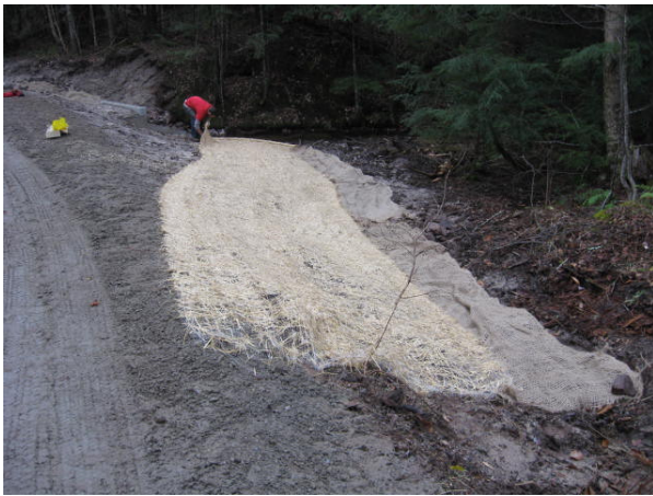
The polymer mixture was spread on all the soil that was disturbed. The polymer not only stabilized the soil but prevents the seed and fertilizer from washing into the stream.
