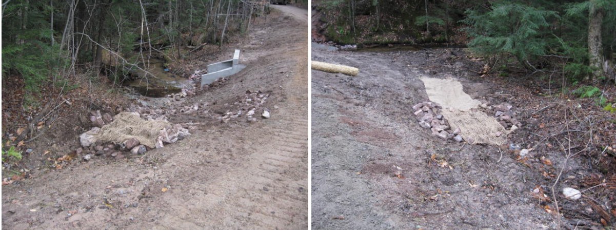
Polymer enhanced rock check systems were installed along the ditch lines.
