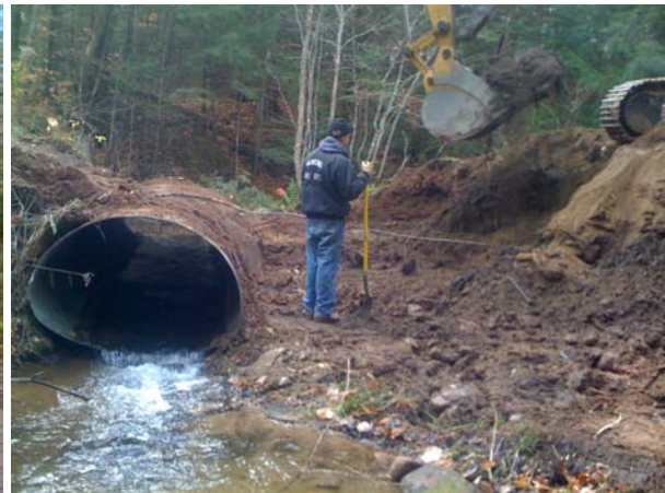
This is the beginning of the removal of the old culvert using an excavator.
