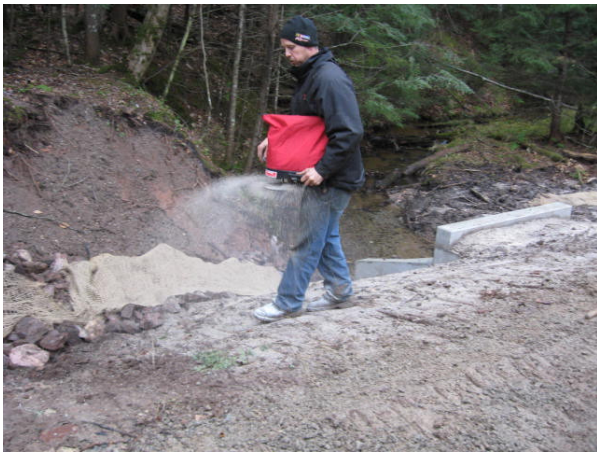
The polymer mixture was spread on all the soil that was disturbed. The polymer not only stabilized the soil but prevents the seed and fertilizer from washing into the stream.
