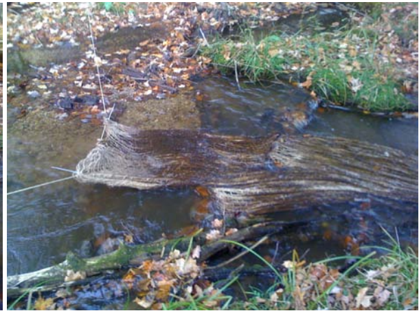
Floc Logs can be seen in the stream preventing turbidity migration.
