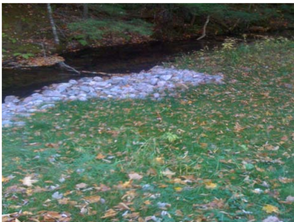
The polymer mixture was spread on all the soil that was disturbed. The polymer not only stabilized the soil but prevents the seed and fertilizer from washing into the stream.
