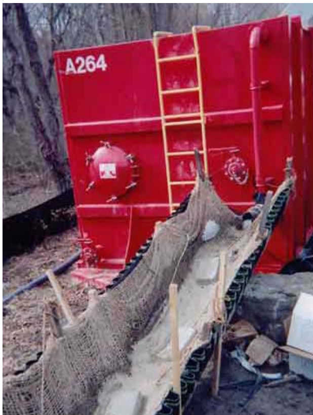
The fractionation tanks acted like settling basins, allowing the heavy solids to settle out before treatment.
